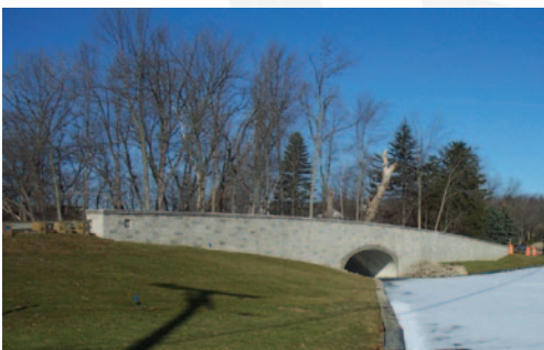
SDA's bridge engineers had to design the Kirkway Bridge in Bloomfield Township to match, in texture and color, the existing stone pillars and walls at the entrance of this subdivision.
